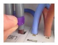
Hold the HCI by its arm and carefully push the HCI onto the Cable Insulation 15 – 50mm from its connection.
